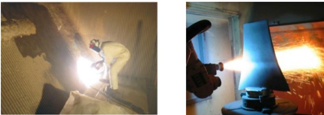
Figure 12. Particle Erosion Coating on Boiler Walls and on Aluminum FDF fans (Energy Production) - Wire Arc Spray, Hard Alloy Coating
